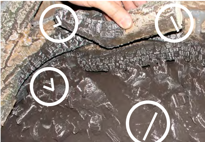
Figure 22 Sec.9 Log 3 installation
