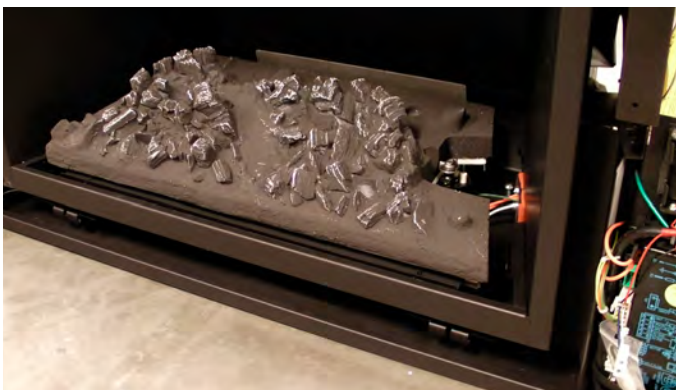
Figure 31 Sec.10 Log burner correctly installed
