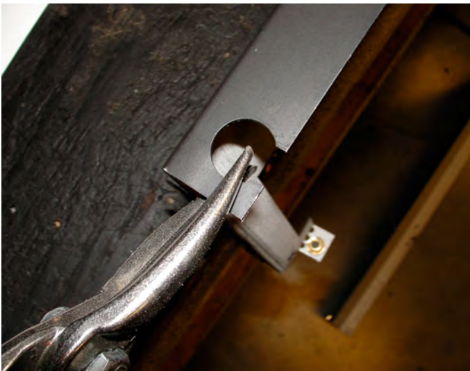
Figure 2 Sec.7 Cutting away excess material
