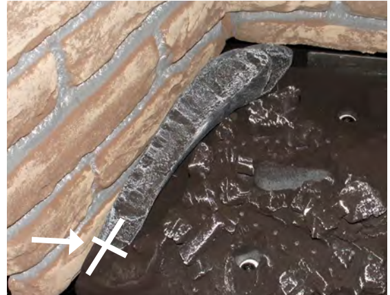
Figure 18 Sec.9 Ceramic baffle installation
