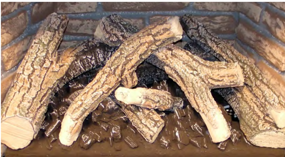
Figure 33 Sec.9 Completed Log Installation
