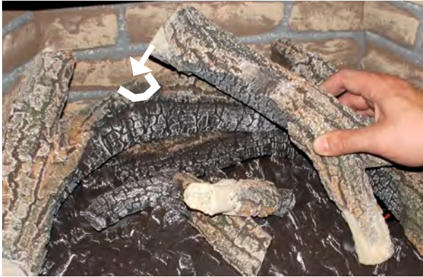
Figure 30 Sec.9 Log 7 installation details
