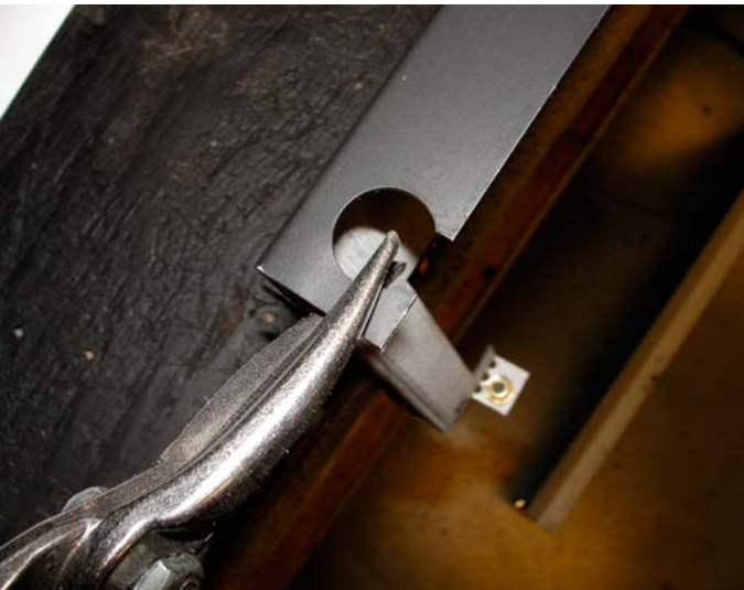
Figure 2 Sec.7 Cutting away excess material
