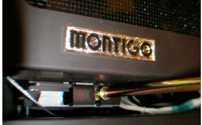
Figure 6 Sec.4 Engaging the Door Tool Into the Door Retainer
