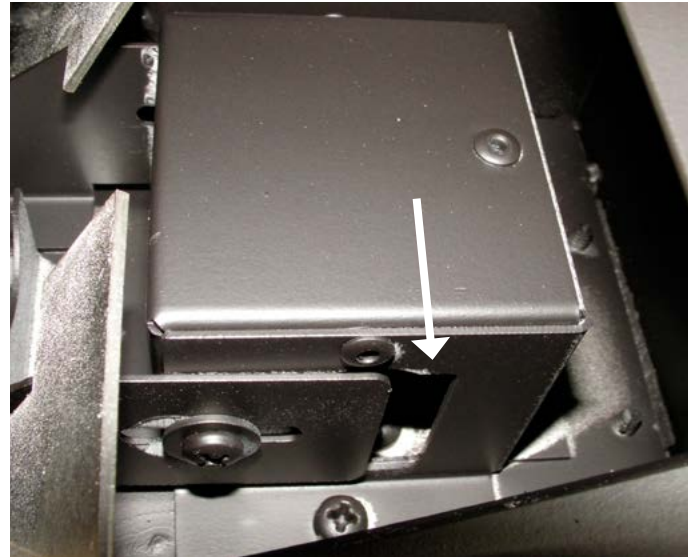
Figure 7 Sec.10 Aeration adjustment opening
