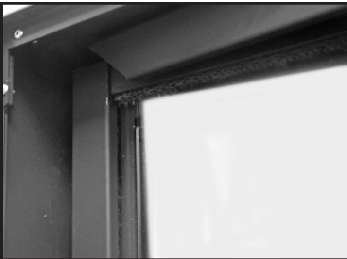
Figure 50: Installing top trim.
