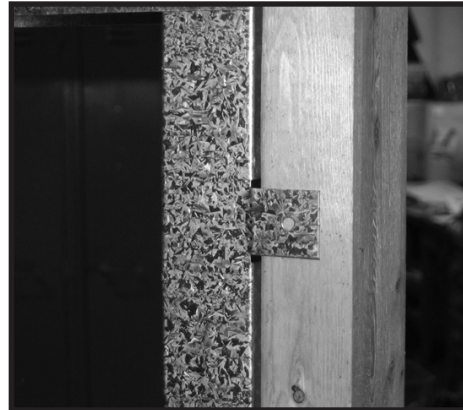
Figure 17: Attaching metal tab to frame.
