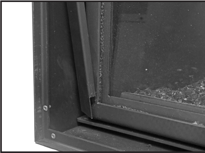
Figure 48: Installing the side trim.
